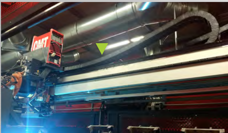
FLEX Modules installed inside an igus® cable carrier with robot mounted on a linear track. Photo courtesy of PA Robotics.
