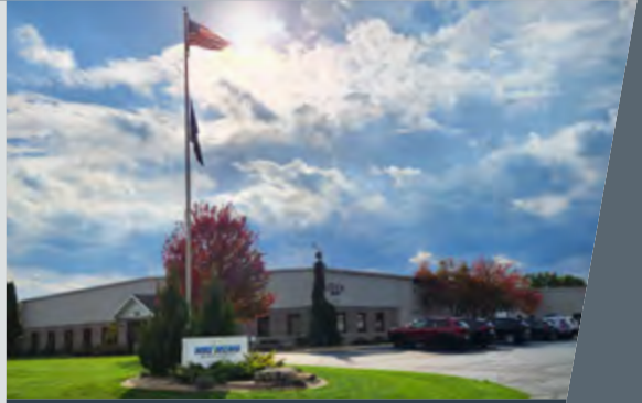
ELCo Enterprises headquarters in Jackson, Michigan
