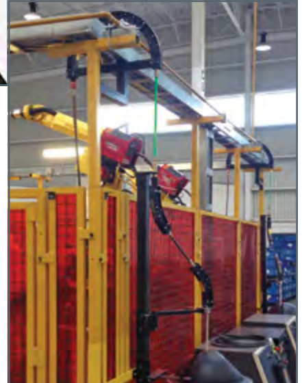
180° Modules installed on cell with two robots and the Non-Stop® Wire Dispensing System
