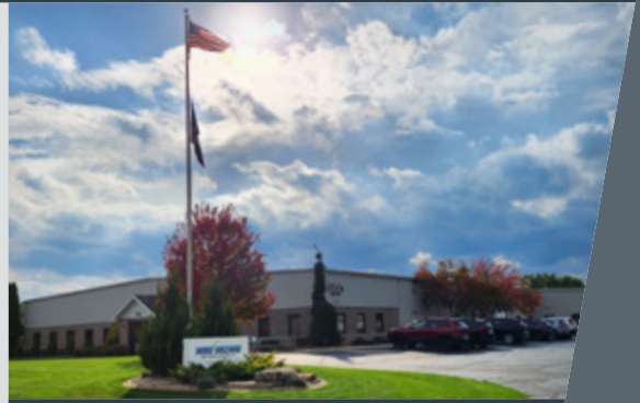
ELCo Enterprises headquarters in Jackson, Michigan
